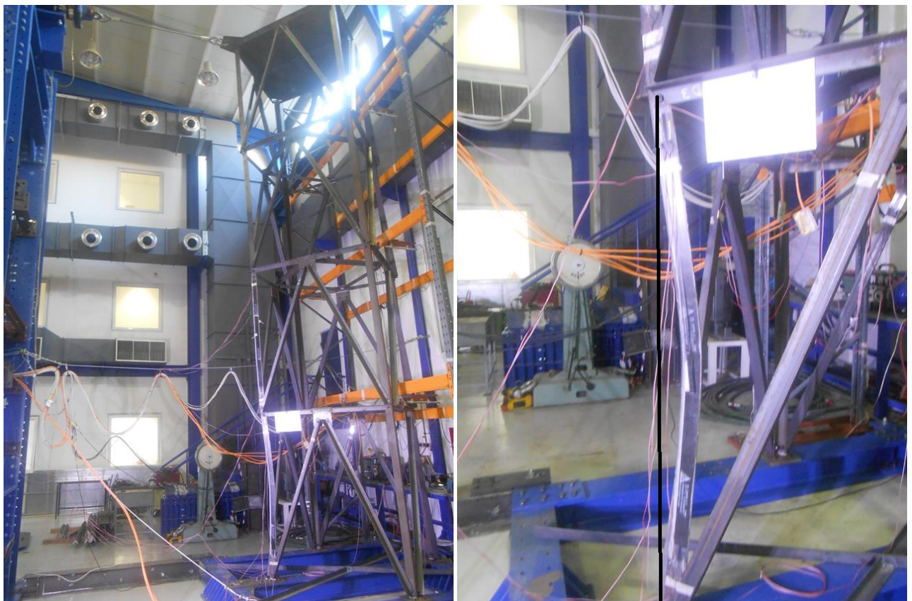
Figure 7.36: Tower D-2S. Weak axis flexural buckling of the compression leg towards the heel
