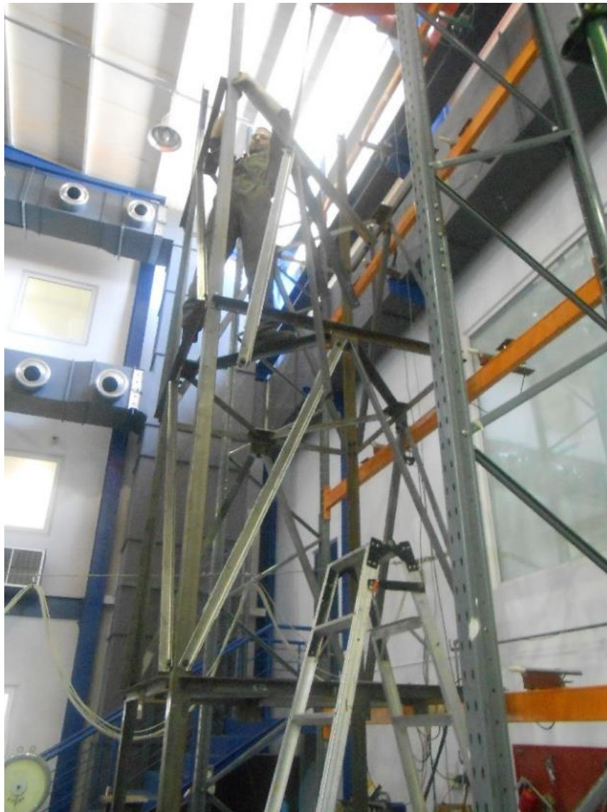
Figure 4.4: Erection of the tower
